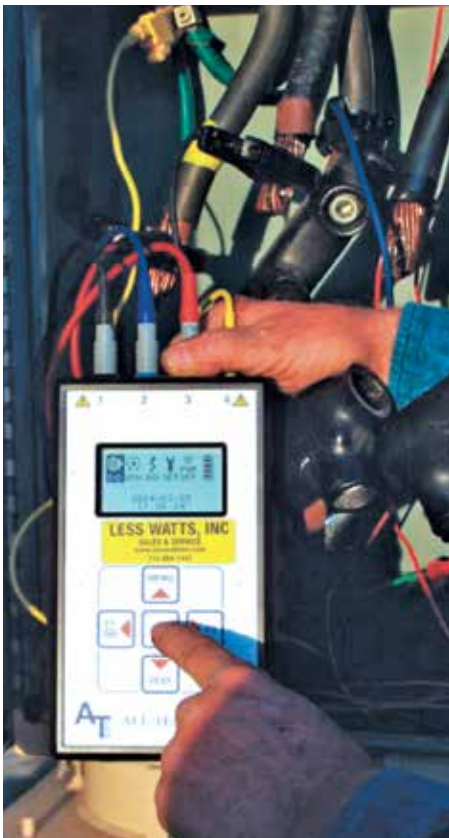
Image 2. Well pump motor tested with the troubleshooting instrument
